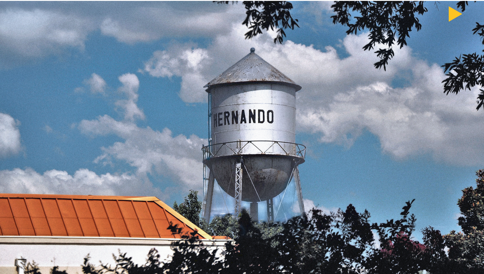
Hernando, Mississippi, built a GIS to track assets, including water towers, water mains and meters.
