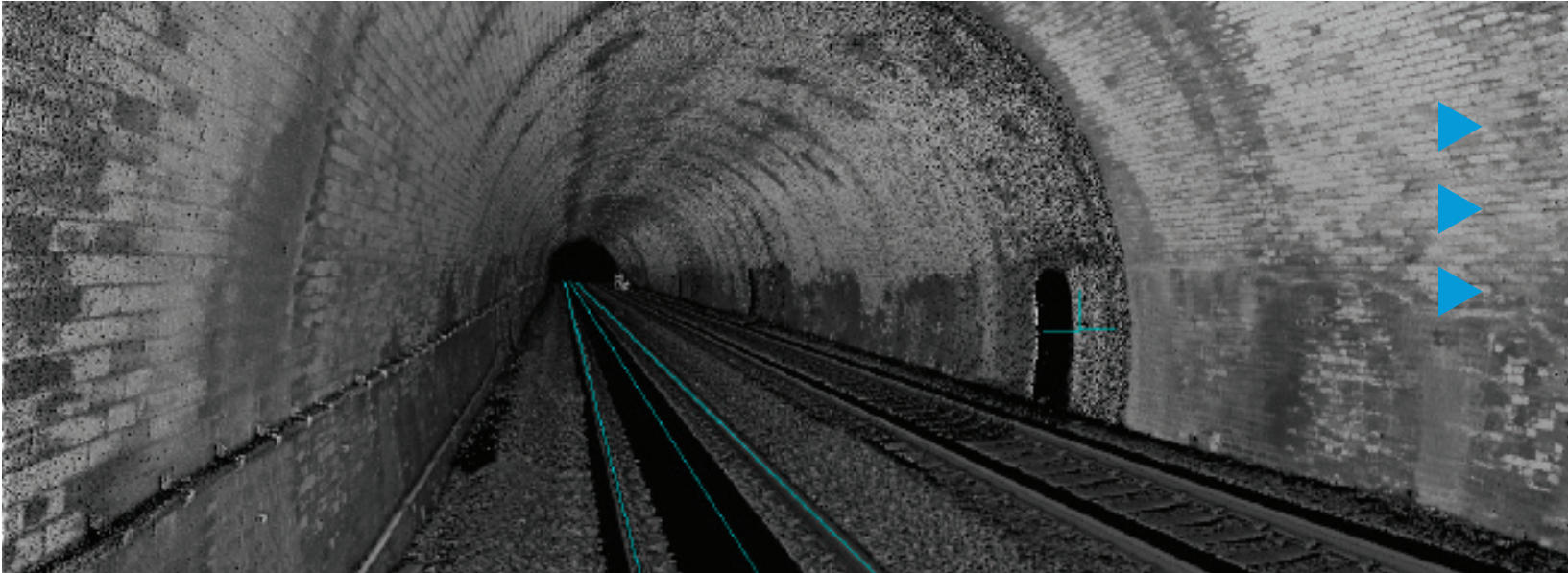
The Trimble GEDO Scan system collects data for track clearance assessment in tunnels
